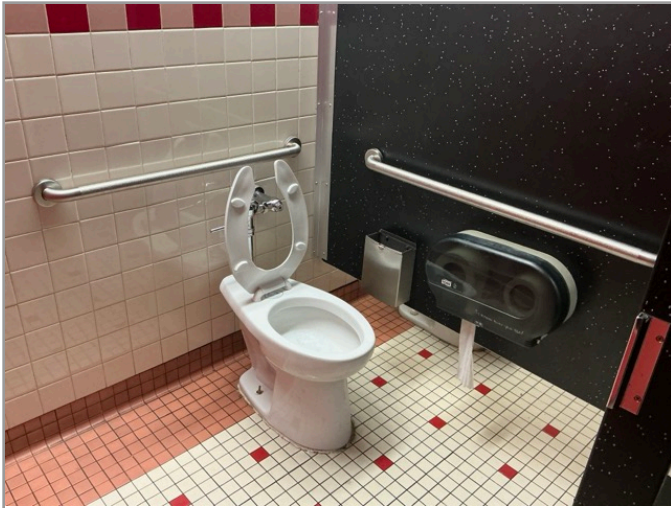
TOILET STALL OVERVIEW
