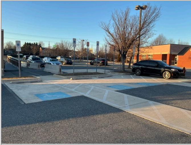
OVERVIEW OF ACCESSIBLE PARKING AREA
