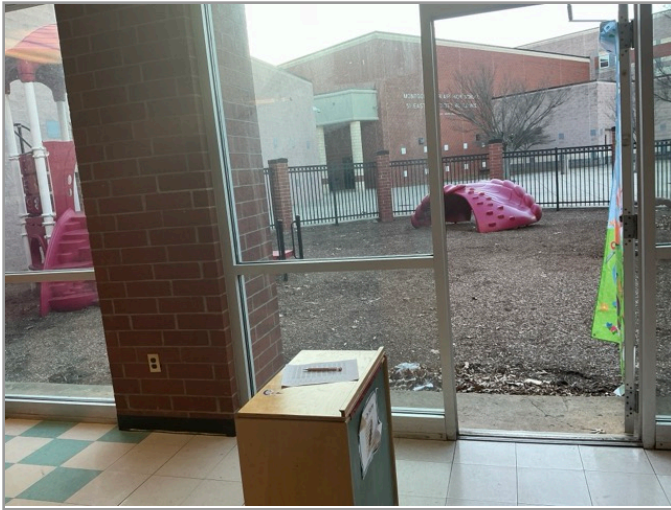
ACCESSIBLE ROUTE TO PLAYGROUND
